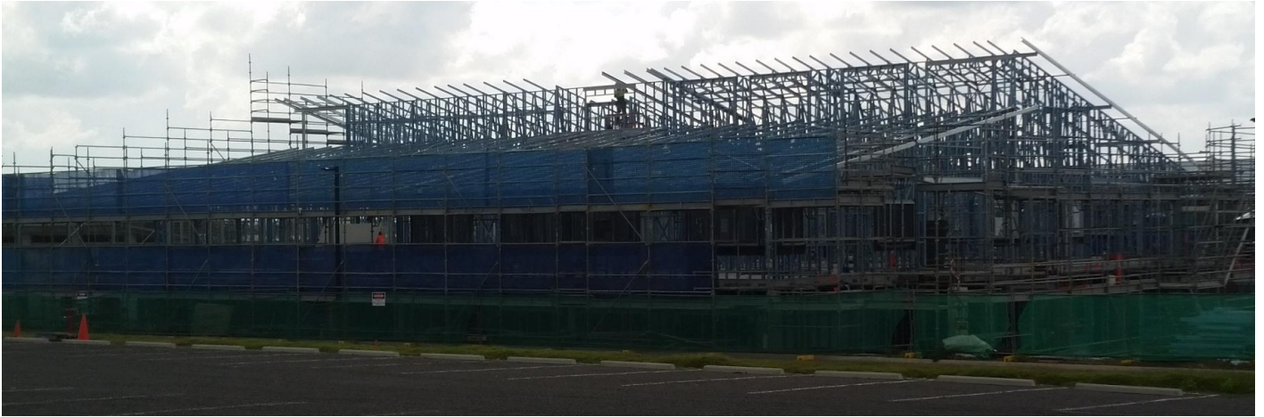
2400m 2 – 2 level – Design & Construct – Light Gauge Steel Framing
