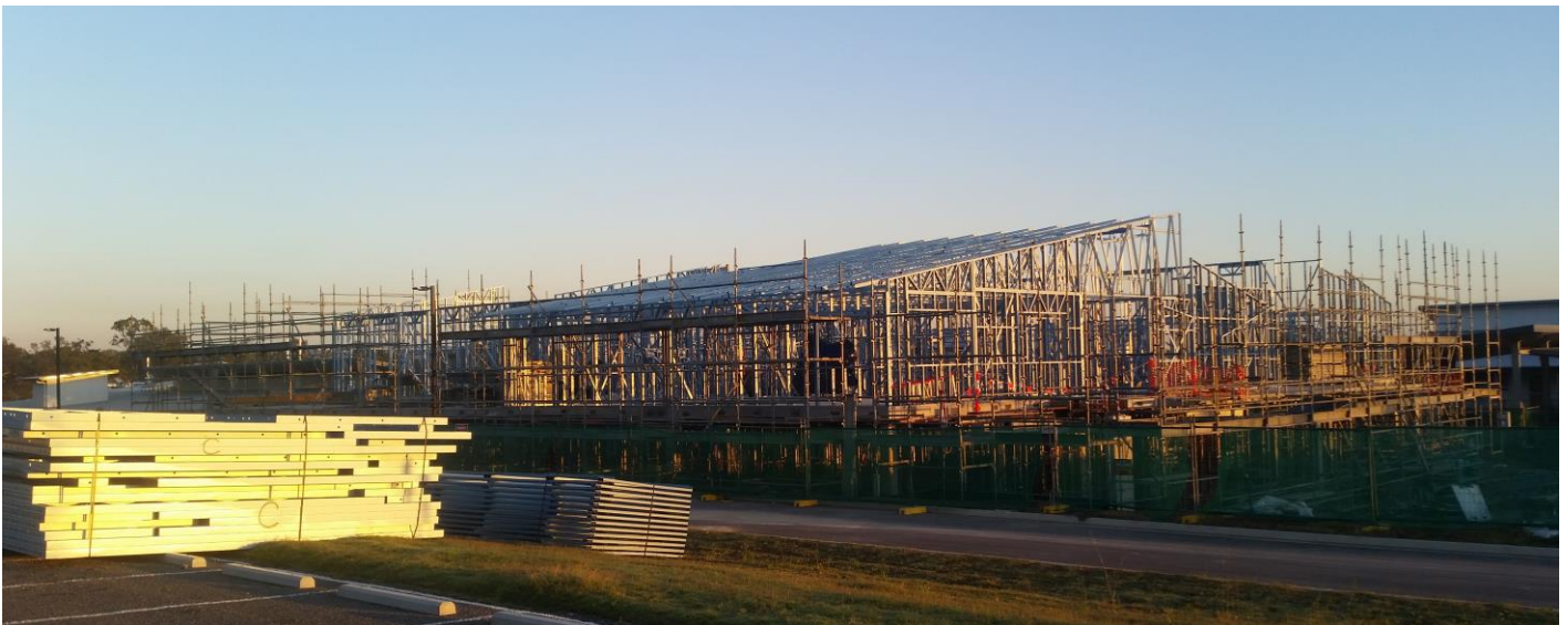
2400m 2 – 2 level – Design & Construct – Light Gauge Steel Framing
