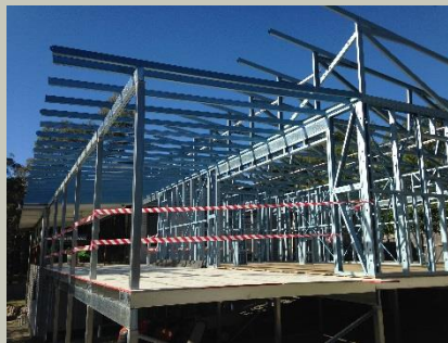
Steel Framed Addition with steel sub-floor System
