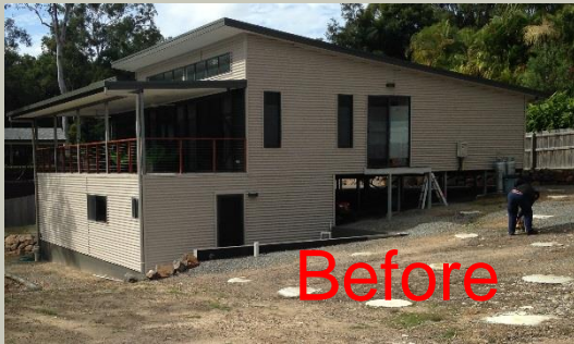
Steel Framed Addition with steel sub-floor System
