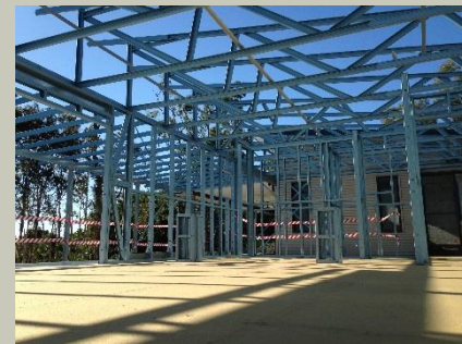
Steel Framed Addition with steel sub-floor System
