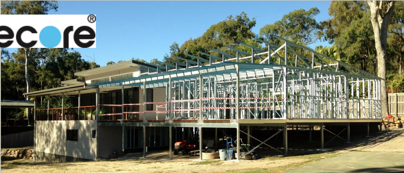
Steel Framed Addition with steel sub-floor System
