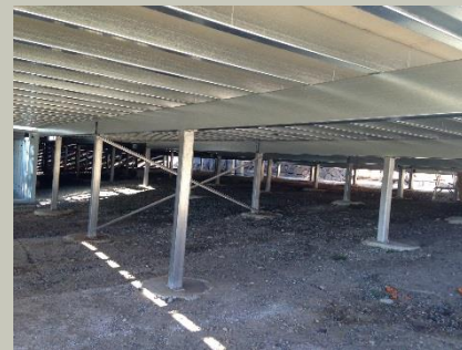
Steel Framed Addition with steel sub-floor System
